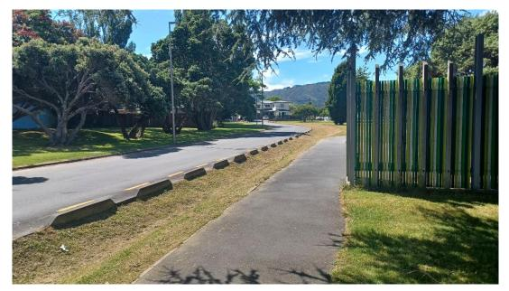
Photo 12 – slotted kerb and swale next to road at Avalon Park, constructed to hold and slow water runoff from the road before it enters the stormwater network.
