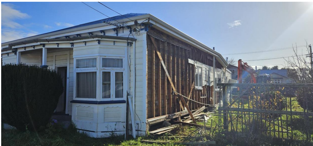
Above images: deconstruction works in progress at Tama Street project. Floorboards and external weatherboards are being removed (by others) to be repurposed elsewhere.
