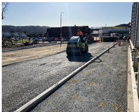
Rear plant year civil works are continuing. Kerb and channel formation are nearing completion.
