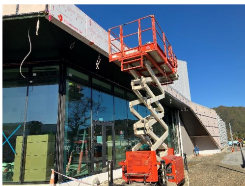
Cladding of the Everest Ave canopy continuing, glazing along this elevation completed.
