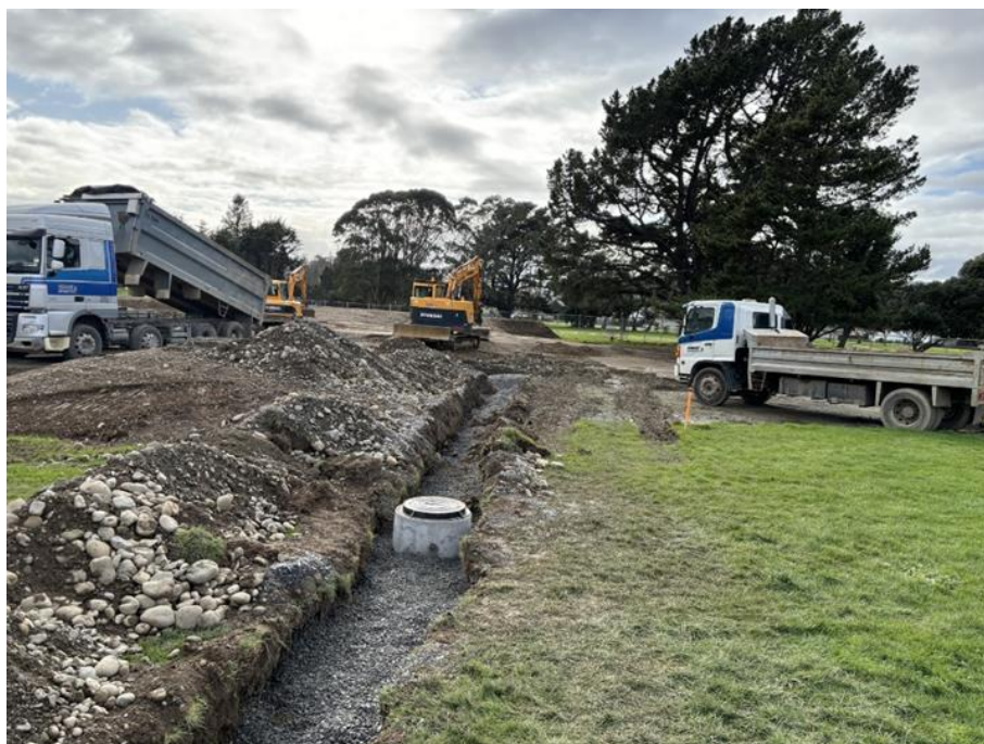
3408- Bubble up sump and trenching for drainage.
