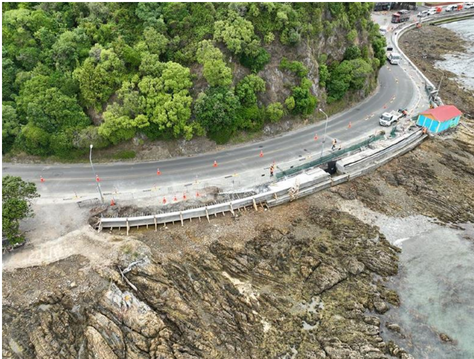
Sorrento Bay Seawall Construction
