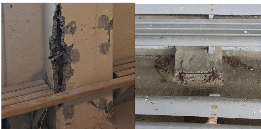
Image 1: Concrete Corrosion and Spalling Petone Grandstand.
