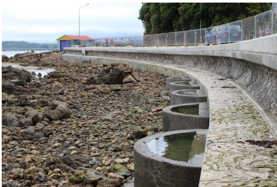
Completed section at Whiorau/Lowry Bay showing tidal pools and ecological designs integrated into the seawalls.
