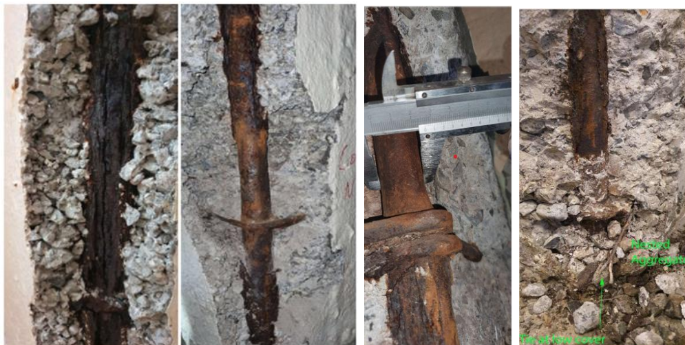
Images 3-6: Severe Corrosion to Reinforcing Bars.
