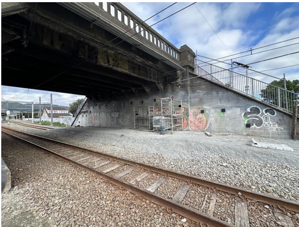
Rail Corridor - Phase 3 anchoring complete
