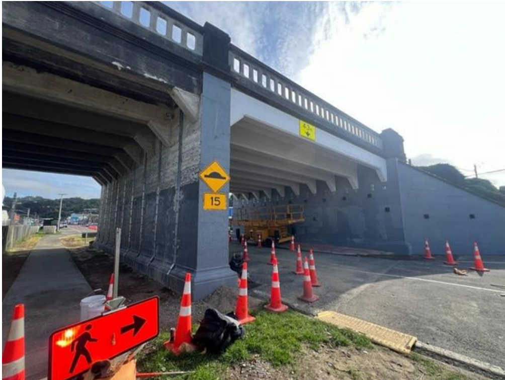
Road Corridor: Phase 1 anchors and Phase 2 linkage brackets are complete
