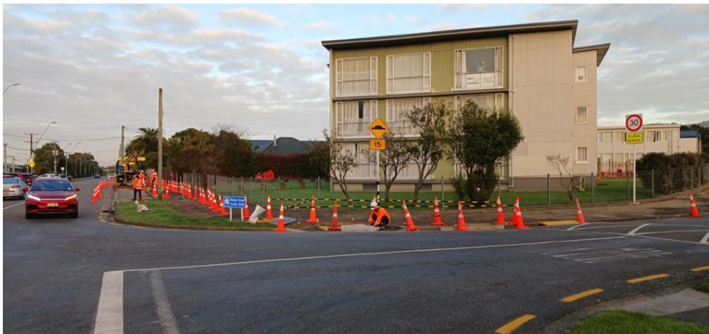
Start of Oxford Terrace Shared Path
