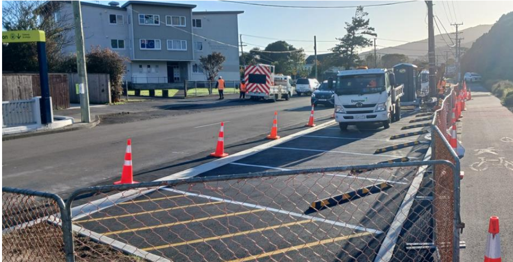
Oxford Terrace Carpark Extension
