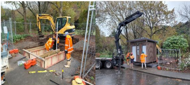
Image 21: Foundation for Belmont Toilet Image 22: Toilet Craned into Place
