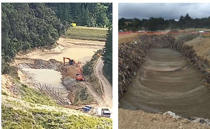
Figure 4: Sediment removal from sediment pond, and sludge pit for removed sediment
